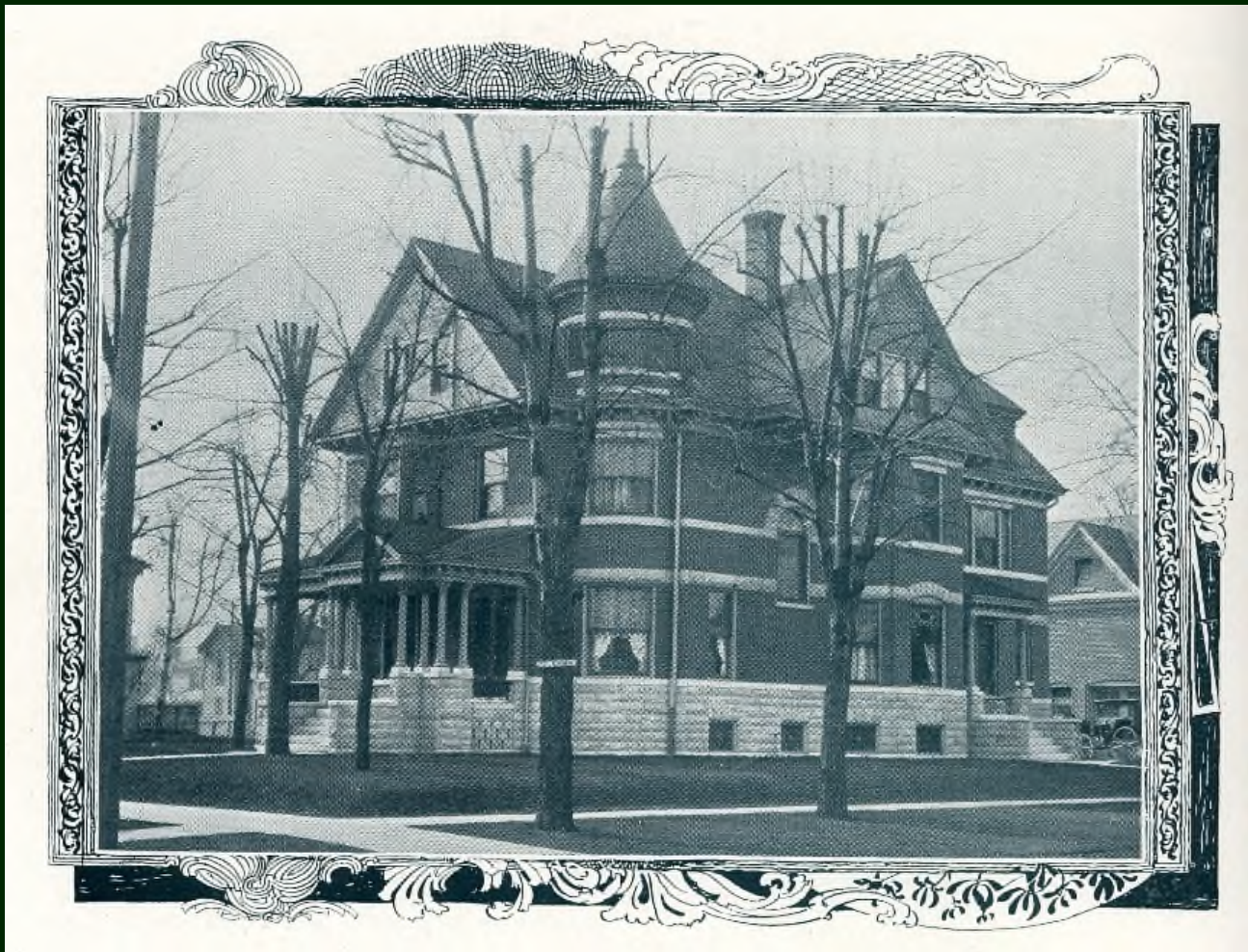
The Joseph Reisch House, 631 N. Sixth Street. Demolished after 1970 ( Illinois Capital Illustrated , Illinois State Journal 1898:116).
